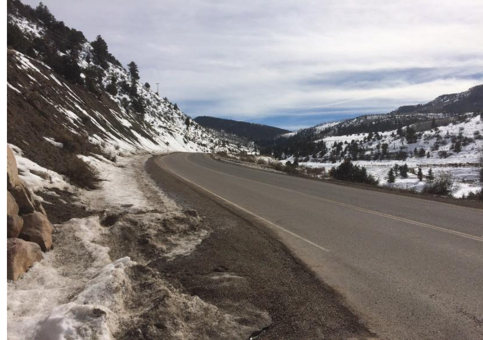
Squaw Creek Road Looking South SD = 880'
