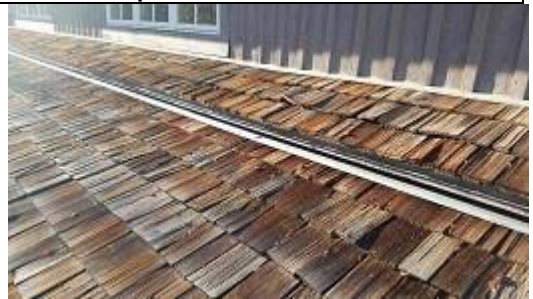
South slope near headwall & vent
