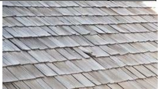
Overview of south slope over pool enclosure
