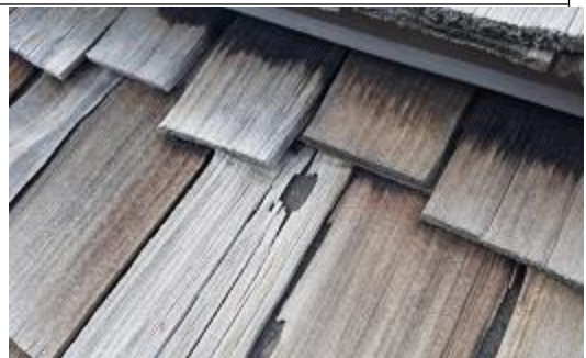
Erosion gaps
