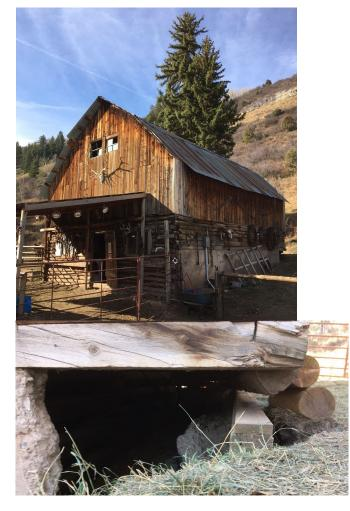
The foundation is <sup>1</sup>/<sub>4</sub> poured concrete and the other <sup>3</sup>/<sub>4</sub> is stacked timber nailed together. Proper design is to stack the timbers and have metal rods in place through all of them to keep them from bowing out and failing.
