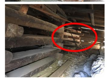
Wire is holding the side walls and roof in place.
