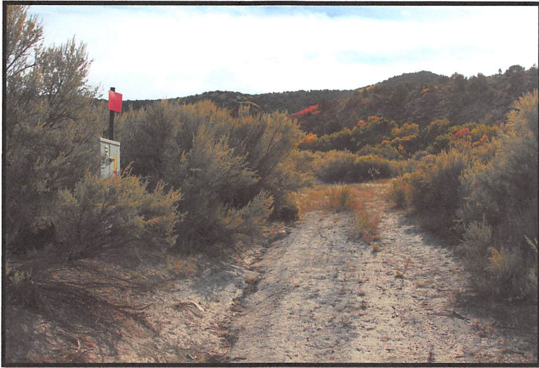
Existing Road. One can easily see that it is not being maintained for emergency access today.
